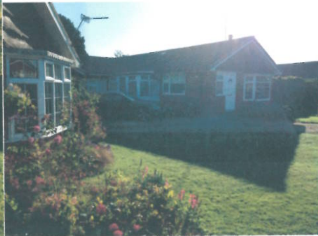
no 30 from no32 driveway – imagine the roof height increasing by another 2.5 metres
